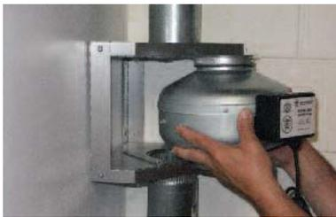
5. Plug fan into Switch It™ receiver and then plug receiver into outlet. Control from anywhere in house with wireless remote.
