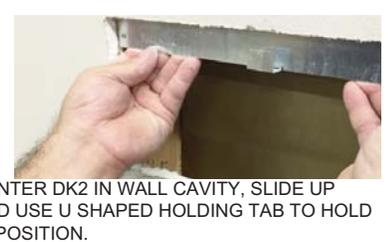
8. Use the U shaped holding tab to temporarily hold the DK2 into position. Use a flashlight if necessary, to verify the small test hole drilled in step 4, (Figure C) lands inside the rectangular AS2 Diffuser opening in the DK2. Adjust accordingly if necessary, (Figure G).
