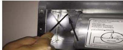
BEND OVER (2) DK2 TABS IN AS2 BLOWER HOUSING WITH A SCREWDRIVER. SECURE BLOWER CABINET TO WALL STUDS WITH (4) PROVIDED SCREWS.
