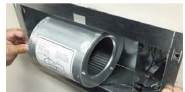
INSERT AS2 BLOWER IN WALL CAVITY OPENING.
