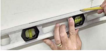
MARK HORIZONTAL LEVEL TOP AND BOTTOM LINES FOR AS2 DIFFUSER.
